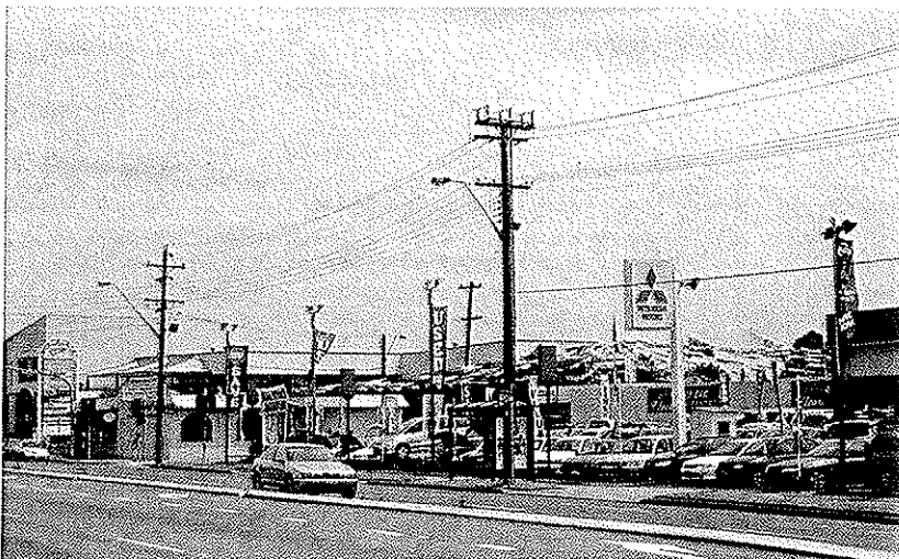
HUME HIGHWAY, LIVERPOOL
